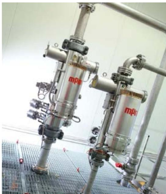
Figure 4: An example for installation of wet gas meters [10]
